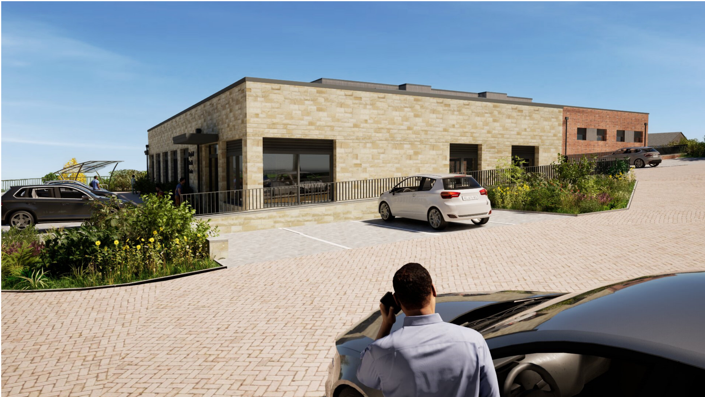
Health Centre West View
