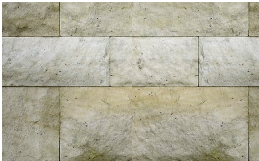
Health Centre Stonework: Wealden Sussex Sandstone
